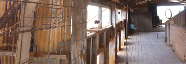
Above Shearing shed at Peron Heritage Precinct.
